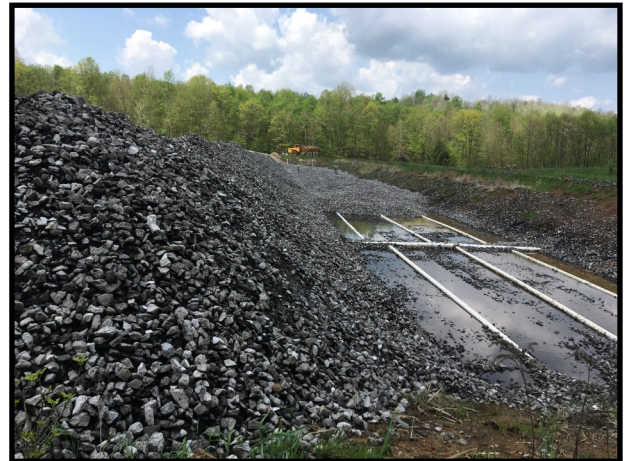
Clogged limestone being removed and replaced at Oven Run Site E
