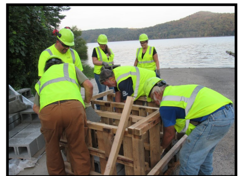
Volunteers construct fish habitat structures
