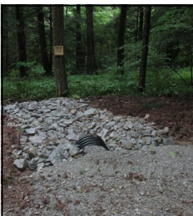
Rip-rap outlet of 18" cross pipe at Shaffer Run Road, Jefferson Township
