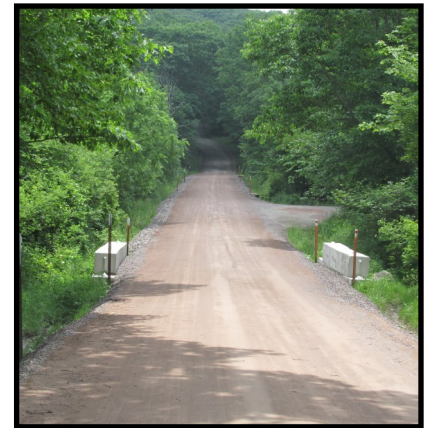
Cranberry Road, Lower Turkeyfoot Twp. Road Fill Project, Dirt & Gravel Road
