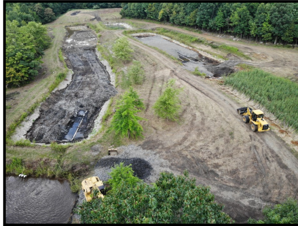
Oven Run System under reconstruction
